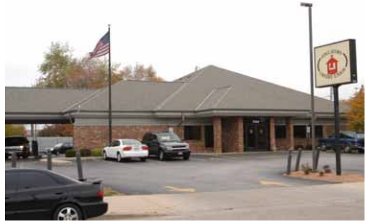
Sound masking is widely used in banks. Lewis has installed dozens of systems in bank branches, including Bank One and Educators Credit Union.
